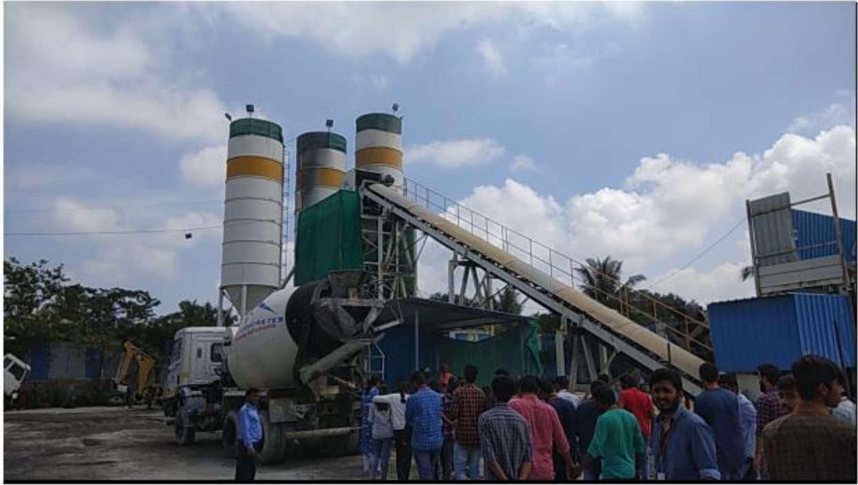
Industrial Visit: Students of Civil Engineering Department,MVJCE attending the process of concrete preparation at “Phoenix RMC Plant” on 04/10/2019
