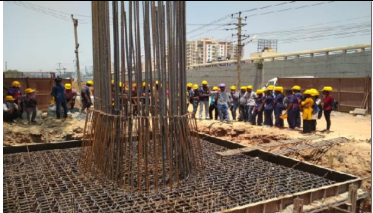
Industrial Visit: Mr. Shishir Kumar, site manager, showing the details of Footing & Reinforcement detailing to Civil Engineering students, MVJCE at BMRCL (Whitefield-Baiyappanahalli Reach-1) Bengaluru on 15/04/2019
