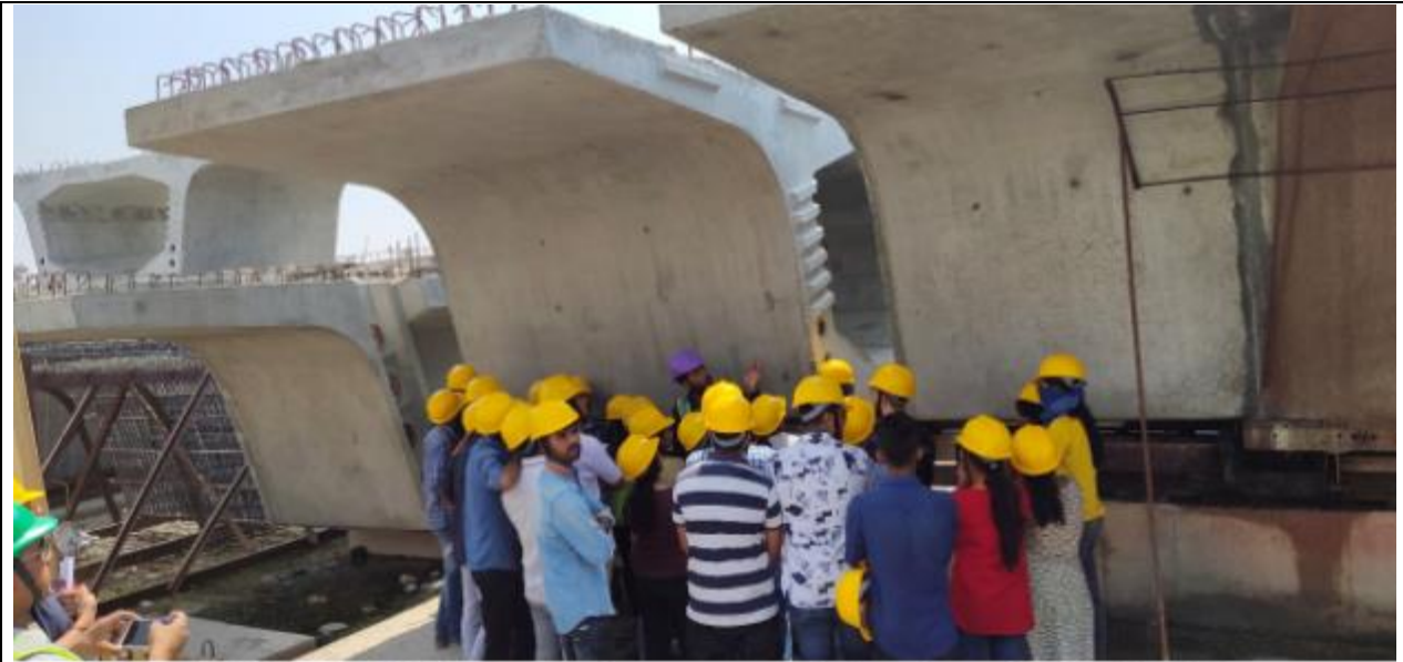
Industrial Visit:Mr.Shishir Kumar,site manager,briefing about the details of site & construction practices to Civil Engineering students,MVJCE at BMRCL(Whitefield-Baiyappanahalli Reach-1) Bengaluru on 11/04/2019
